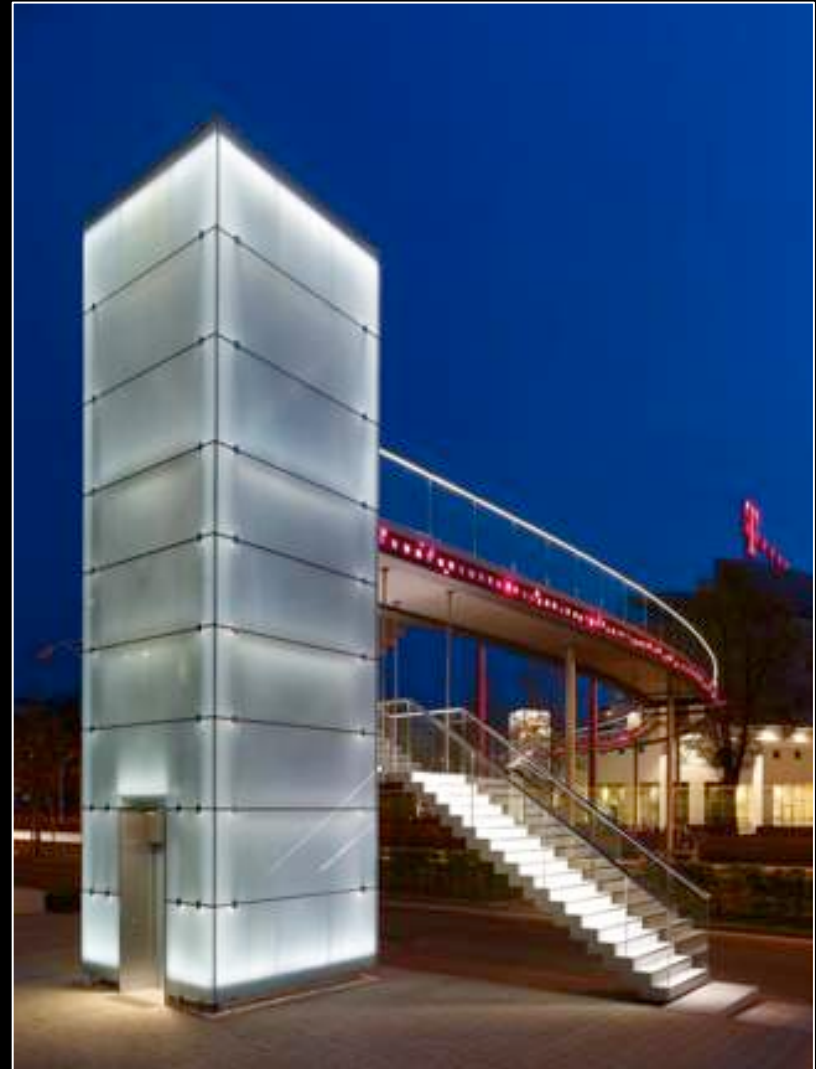
Telekom Bridge, Bonn (Alemania)
